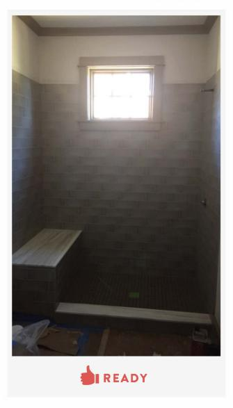
Shower tile is completely installed and ready for glass measurements.
