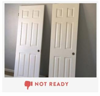
Doors are in the home, but not hung, and cannot install locks or hardware to ensure proper catch and close.
