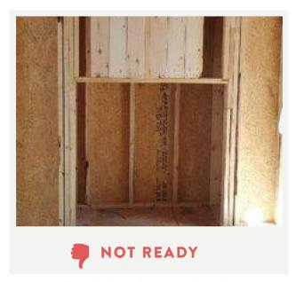
No insulation in chase on exterior walls
