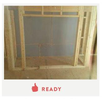
Insulation and air barrier installed
