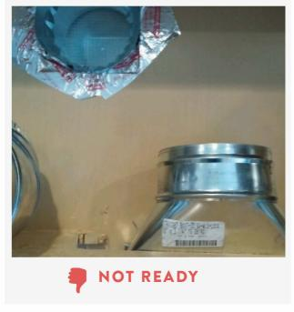
Microwave vent pipe not installed centered
