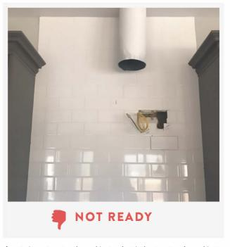
A vent pipe not centered on cabinets, electrical not centered on cabinets
