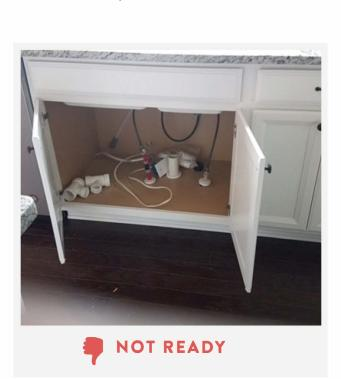
No drain installed for dishwasher
