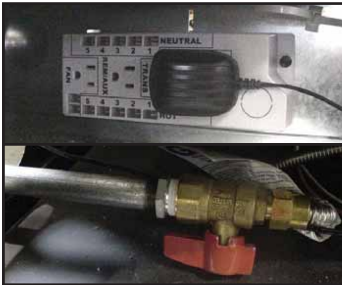
Figure 13.1 Preparation to Install Splatter Guard
