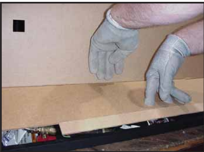
Figure 13.8 Opening Lower Access Panel
