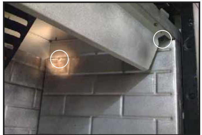
Figure 3.6 Top Screws For Metal Refractory
