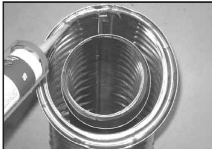
Figure 10.1 High Temperature Silicone Sealant
