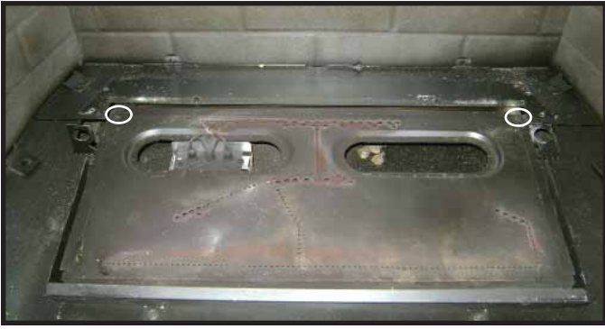
Figure 3.8 Remove Screws from Burner Assembly Rear Corners
