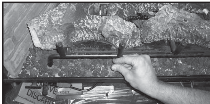
Figure 14.4 Placement of Vermiculite
