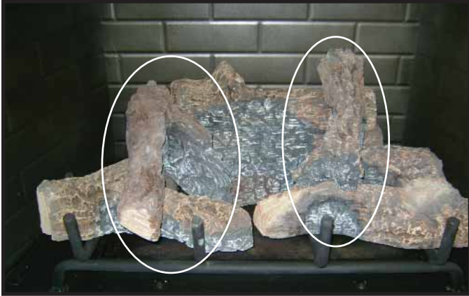
Figure 3.2 Remove Top Two Logs
