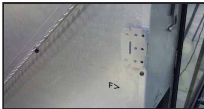
Figure 6.3 Side Nailing Tab in Shipping Position
