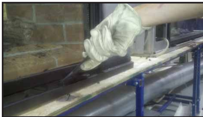
Figure 11.3. Inserting Glass Clip Tool
