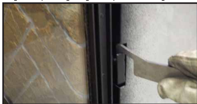
Figure 11.7. Securing Side Glass Clips
