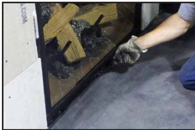
Figure 11.8. Securing Bottom Glass Clips
