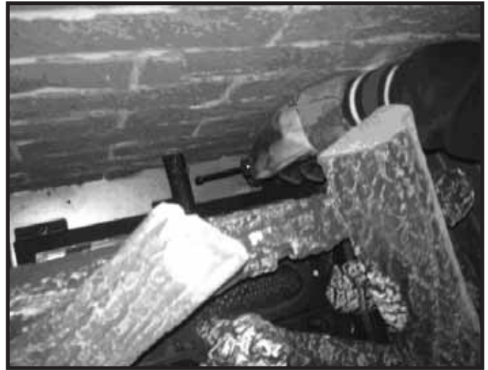
Figure 1. Air Shutter Location
