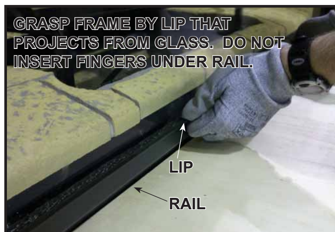
Figure 11.6. Installing Glass
