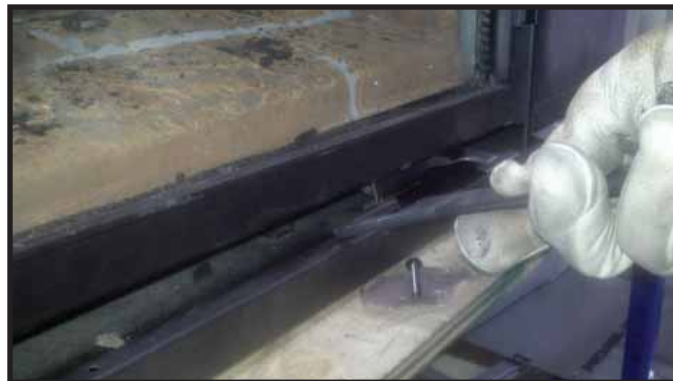
Figure 11.2. Glass Clip Tool Location
