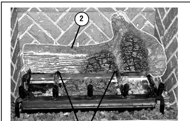
Align Groove At The Bottom Of Log (2) Over The Grate And Push It Towards The Rear.
