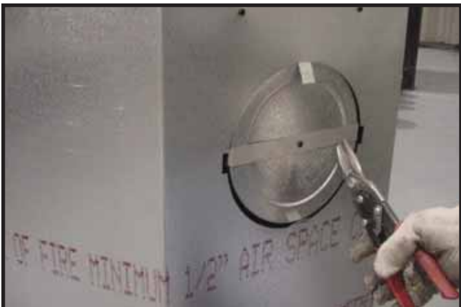
Figure 9.8 Cut the metal retaining band and fold the sides out.
